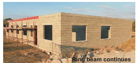
Internal walls and ring beam in July
