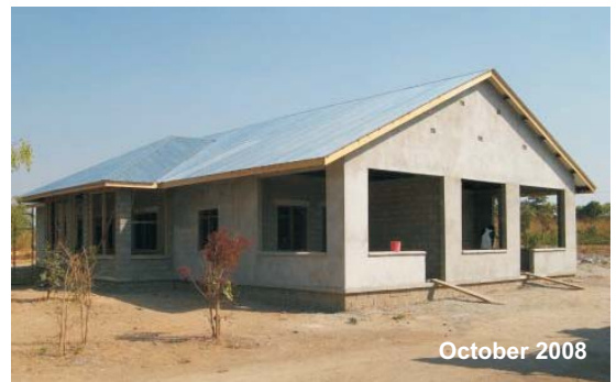
Topping out, end of September 2008
