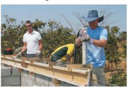
spreads the load of the roof along the walls. Shuttering was assembled in order to pour the concrete in sections and this was
