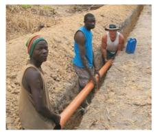
continuing to the septic tank located at the bottom of the site. The installation of the pipes, manholes and rodding points was overseen by Paul, one of the group of Brass Tacks volunteers out to help us in August.
