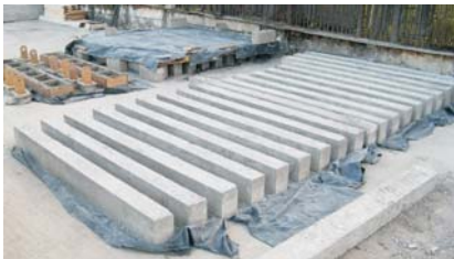
Completed Lintels and Airbrick blocks
